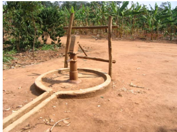
Figure 9: An Abandoned Dry Borehole in Masaka in 2005
